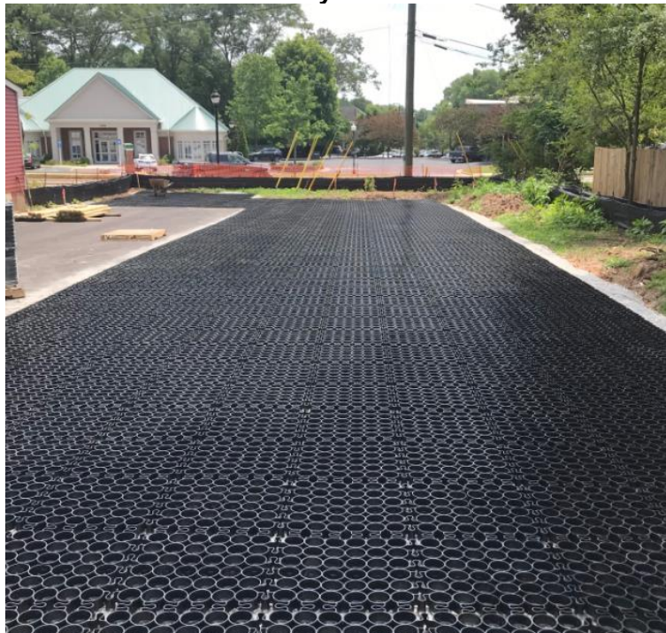
Figure – 3 True-Grid Paver System Prior to Gravel
