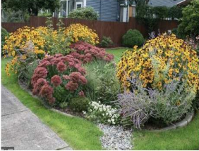
Figure 10. Bioinfiltration with cobble inlet.
