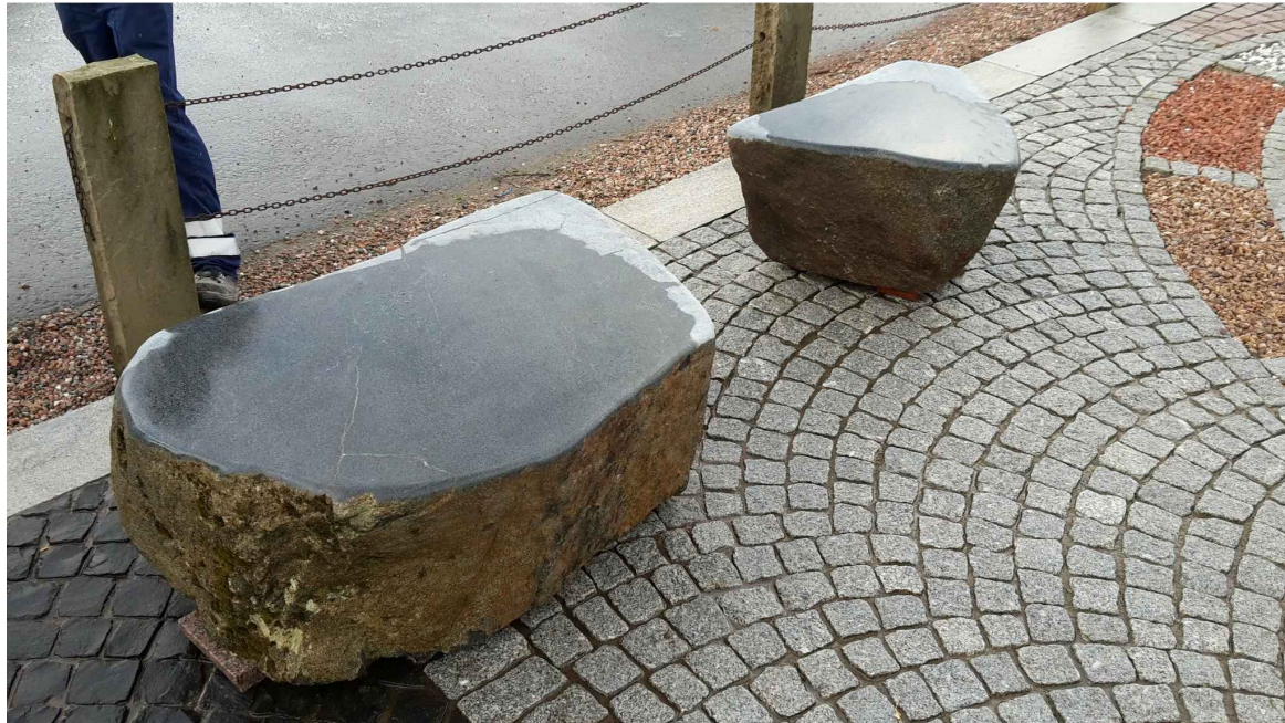
BOULDER TO BE GRANITE. TOP OF BOULDER TO BE REFINED BY LOCAL STONE MASON.
